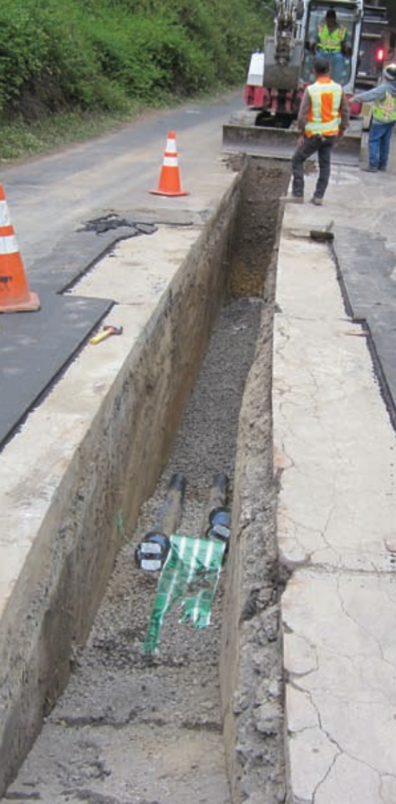
Force main replacement on Cannon Drive
